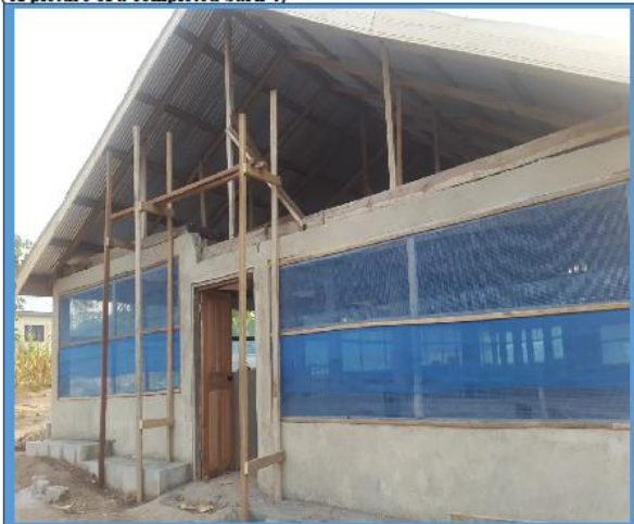
(A picture of a completed barn 4)
